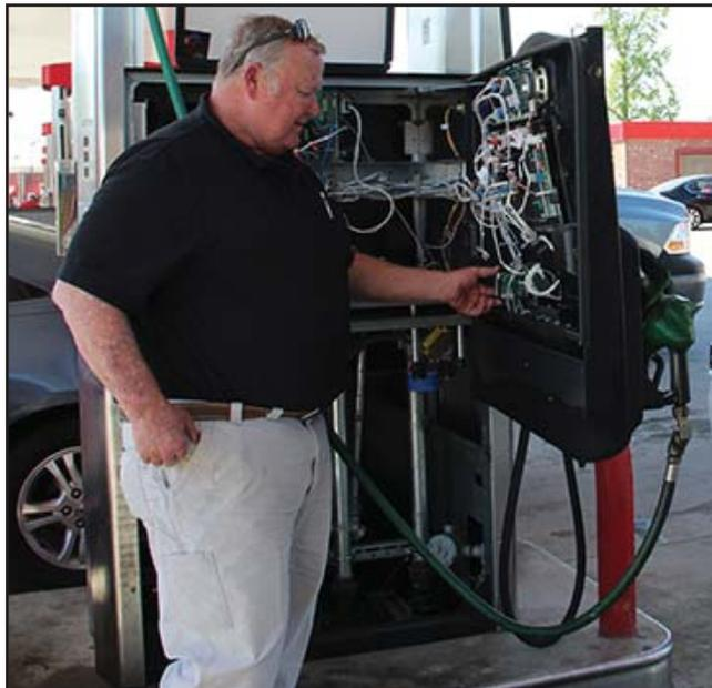
An NCDA&CS Standards Division inspector checks a gas pump for a credit card skimmer.
