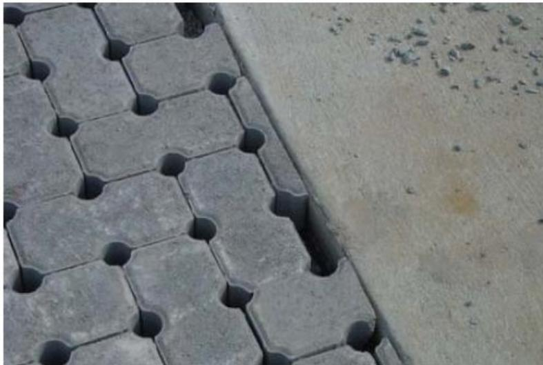
**Figure 10.5 Pavers abutting a concrete edge.**
