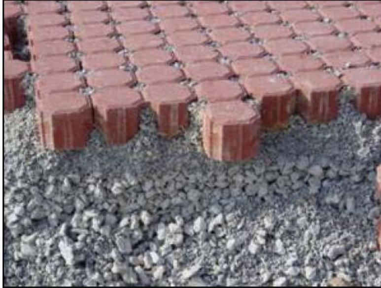
**Figure 10.6 Gravel layers under permeable pavers.**
