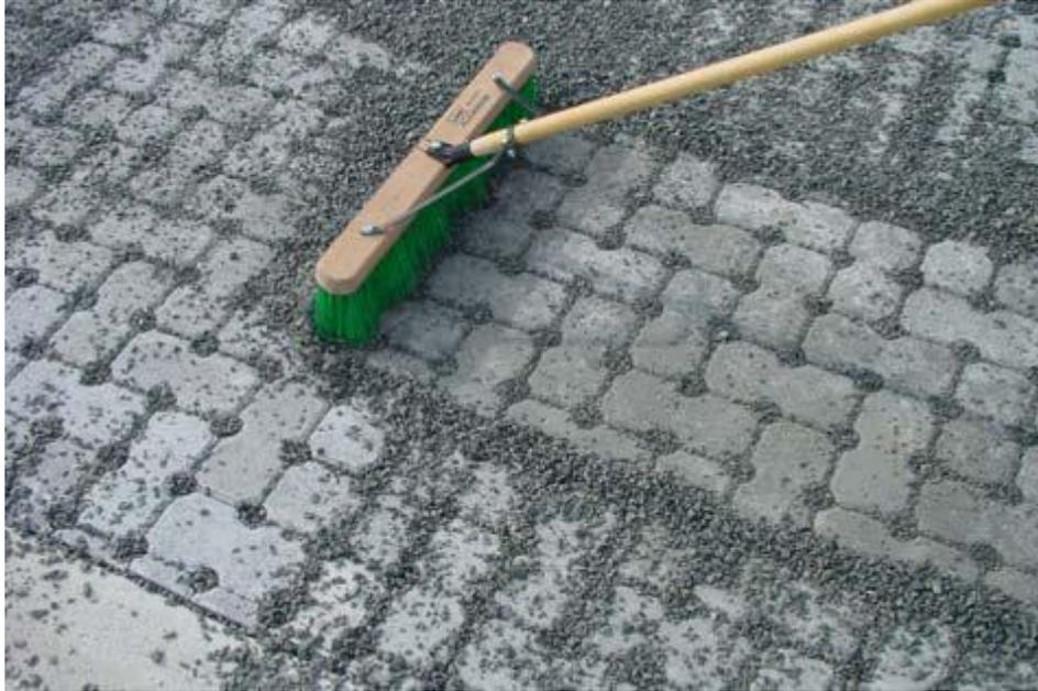
**Figure 10.7 Filling permeable paver voids with gravel.**
