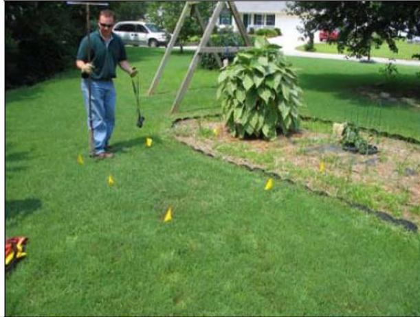
Figure 6.5 Mark wetland area prior to excavating the area.
