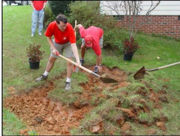
Figure 6.7 Berm construction at downslope edge of BMP.
