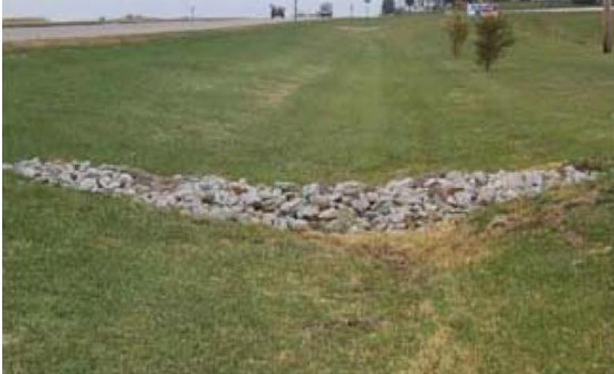
**Figure 6.4 Swale with check dam constructed of stone.**
