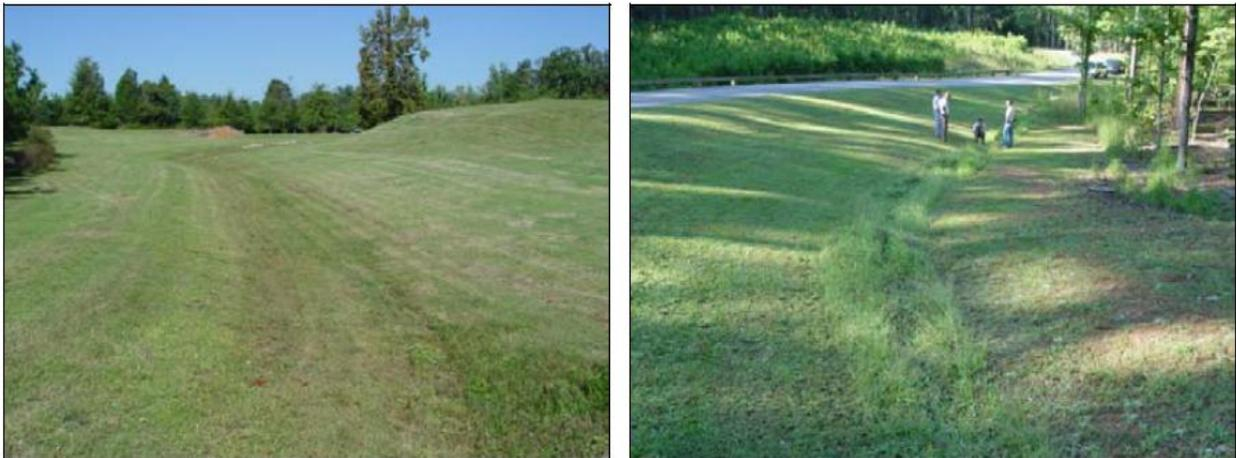
Figure 8.1 shows two swales in the Raleigh-Durham area. Both have turf reinforcement mats. The former is mowed while the latter contains a taller grass stand.
