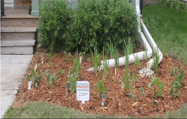
The mulch used here is too large (single-shredded hardwood instead of triple-shredded) and will lead to flotation, likely floating out of the garden. The downspouts will add to this problem. The size of the garden also appears to be less than the treatment volume needed
