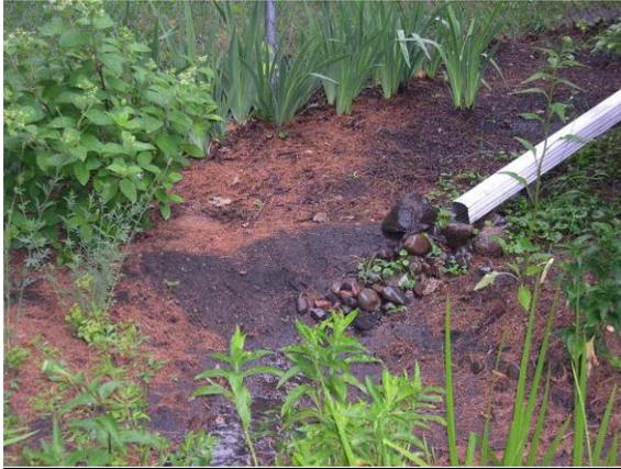
The gutter downspout has concentrated flow at the outlet. The small rocks are not enough to dissipate the energy of the water coming from the downspout and will lead to erosion and sediment.
