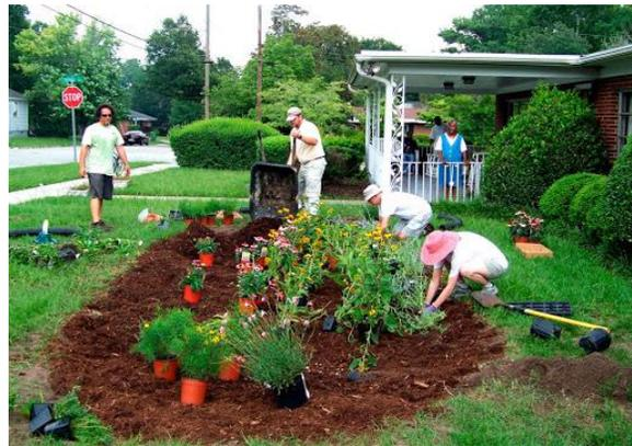
Nearly completed rain garden with a good layer of proper mulch and plant material selection. As this is not quite completed, any areas of heavy mulch layers (such as at the forefront of the photo) can readily be raked out for the proper, consistent layer.
