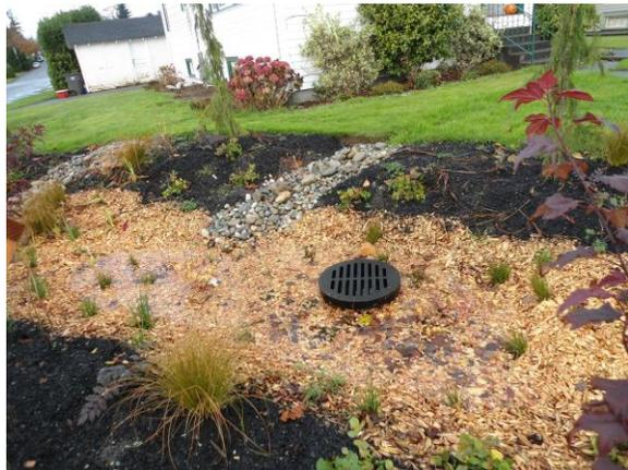
The vegetation is minimal on this site. While newly planted and immature, even when fully grown the spacing for this garden is not optimal. Care should also be taken on the cobble drainage coming into the garden for potential erosion and sedimentation. Note the mulch, it is too coarse and will likely lead to flotation, potentially filling the drop inlet (the black grate in the center) with debris.
