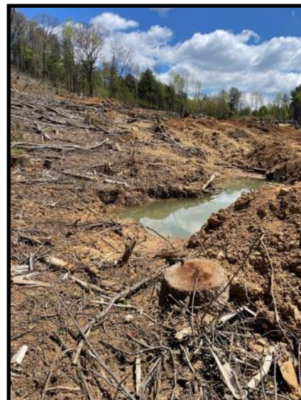
BMPs being implemented on a timber tract in Western North Carolina. Left: trench along a skid trail to direct run off to a stable outlet. Right: sediment catch pit.
