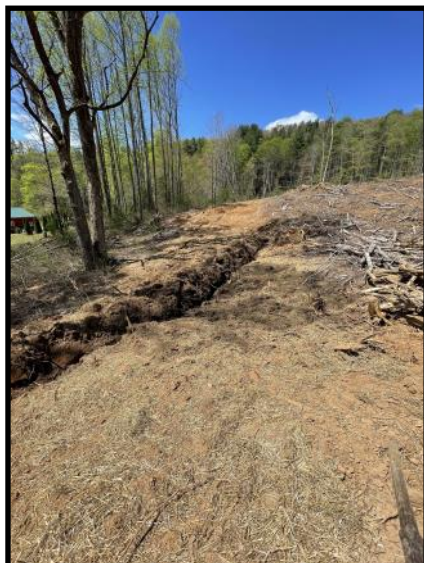
BMPs being implemented on a timber tract in Western North Carolina. Left: trench along a skid trail to direct run off to a stable outlet. Right: sediment catch pit.
