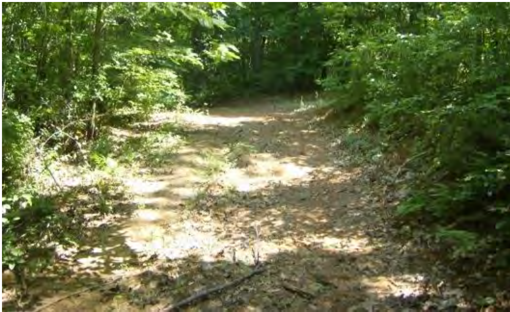
Figure 7D: A forest haul road with the lowest road standards of the examples shown Picture note: Compared to the previous three examples, this road is narrower, heavily shaded, and partially covered by leaves, sticks and other organic debris. Traffic volume is infrequent and therefore does not need as many BMPs to provide similar water quality protection to the other examples. Assuming the remainder of the road is stable and future access is not needed, it is best for water quality protection to allow the road to naturally recover.
