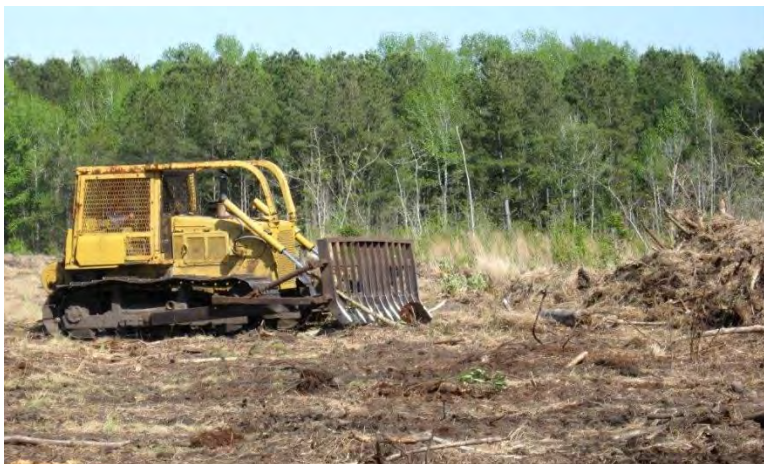
Figure 9E: Bulldozer with a toothed root rake piling debris
