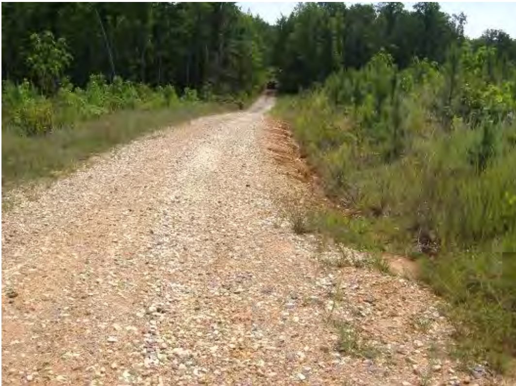
Figure 7B: A forest haul road with lower road standards than figure 7A Picture note: Compared to 7A, this road is narrower, has more bare soil, fewer water control structures, and steeper grade.
