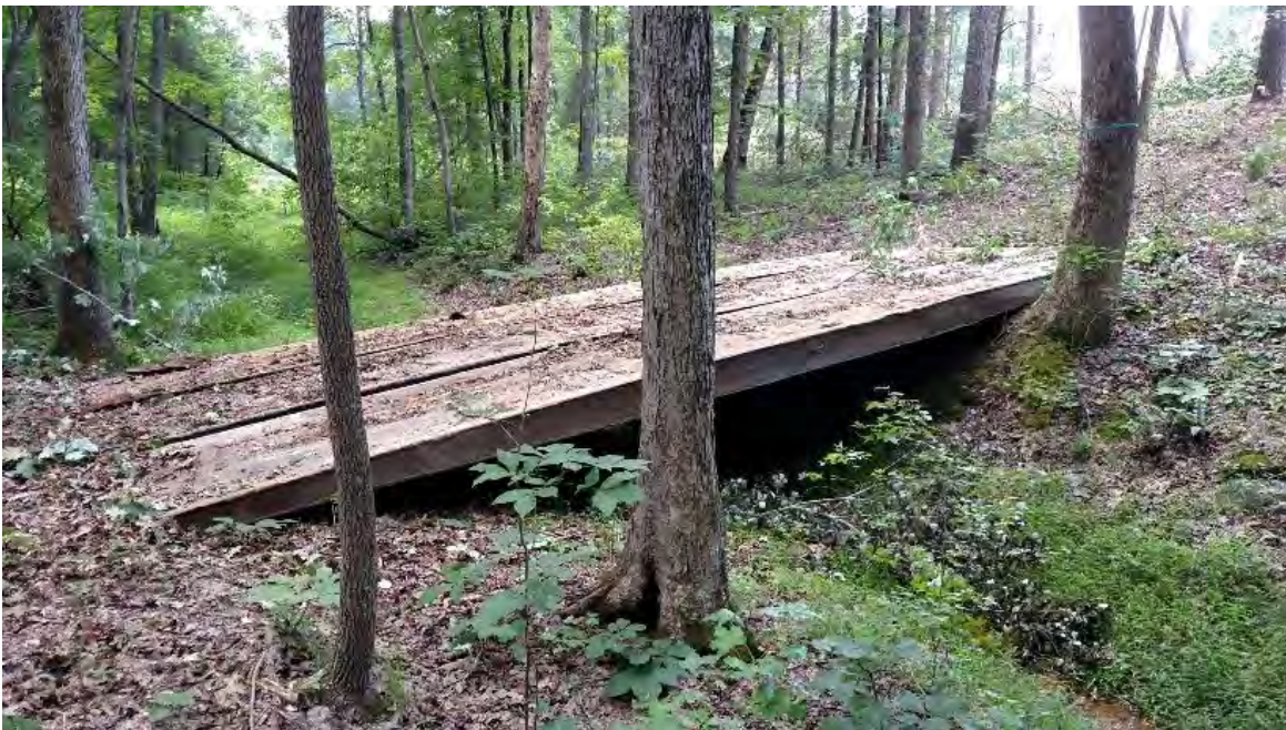
Figure 6B: Example of a temporary steel bridgemat stream crossing
