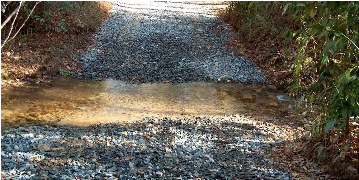
Figure 6L: A newly renovated and improved ford crossing
