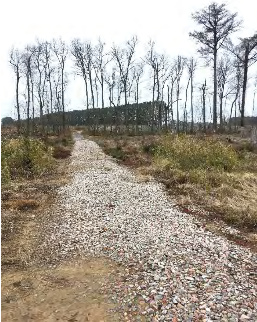
Figure 8C: A forest road constructed through a wetland
