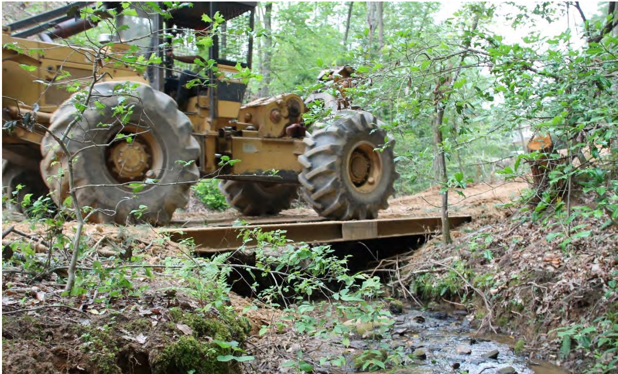
Figure 6G: An example of properly installed steel bridgemats
