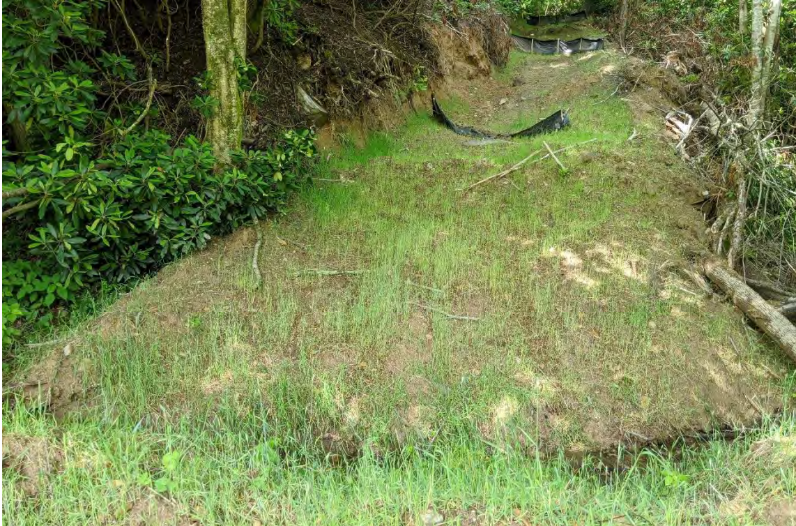
Figure 10A: Stream crossing after completion of logging
