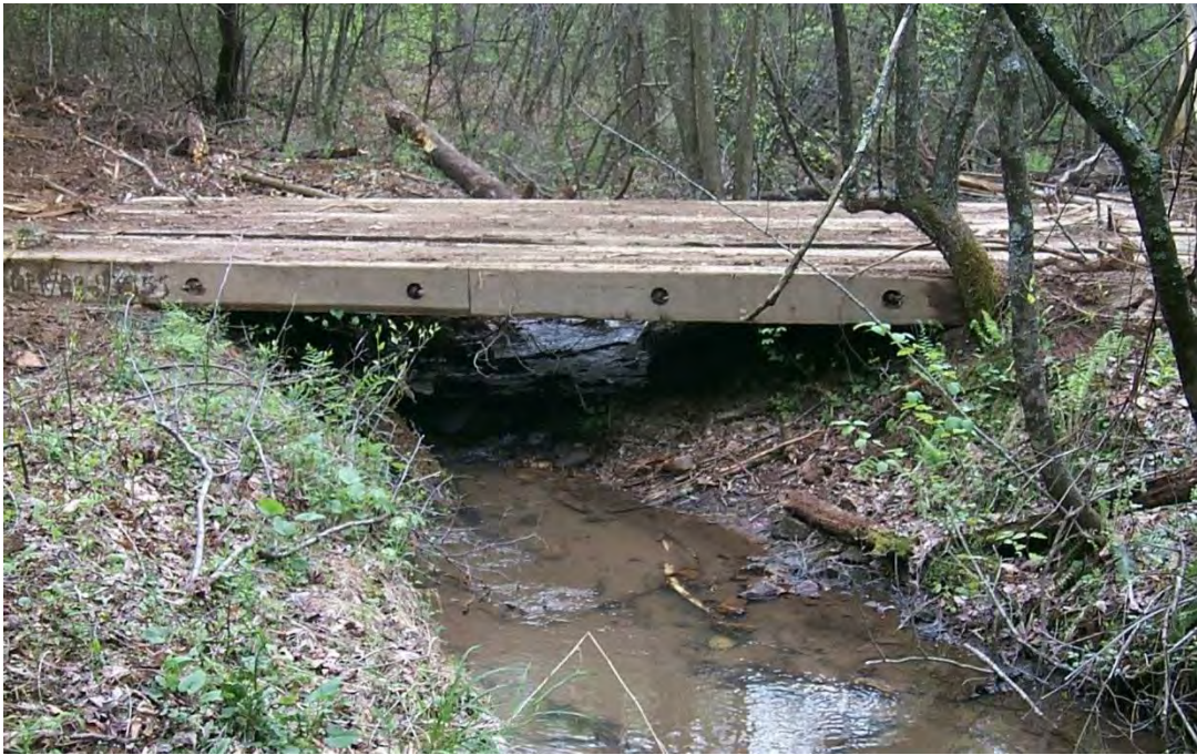
Figure 6F: Side view of a wooden bridgemat skid trail crossing
