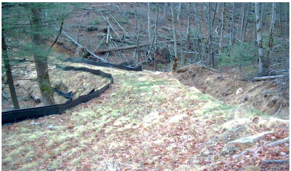
Figure 10B: Stabilized skid trail in the mountains
