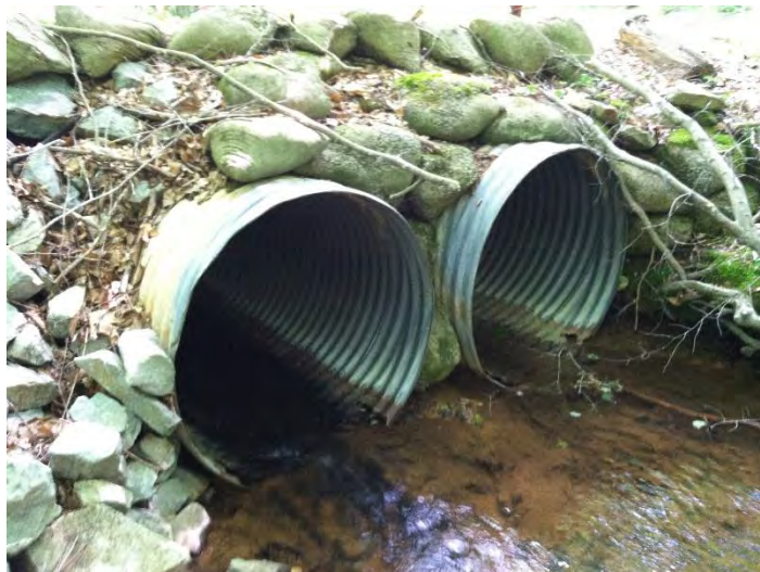
Figure 6-1: Culverts installed for a forest road stream crossing
