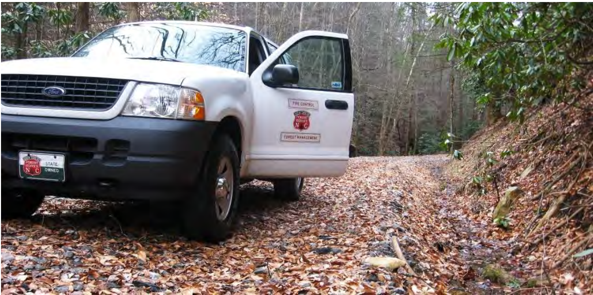
Figure 5H: A forest road with a shallow inside ditchline
