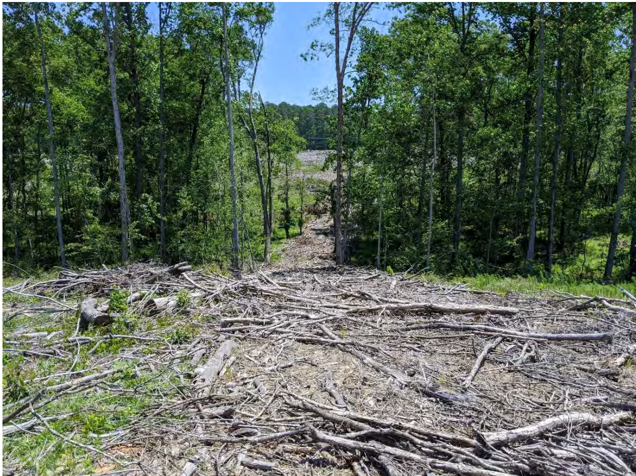
Figure 10D: Primary skid trail stabilized with abundant logging slash
