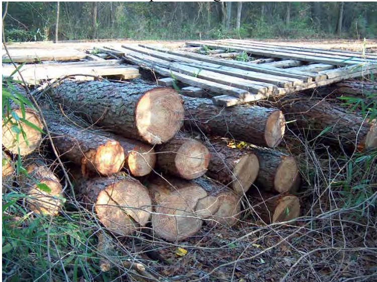
Figure 6H: A pole crossing installed within a dry ditch for temporary log road access Picture note: This pole crossing uses adequately sized logs to provide support and are free of soil, limbs, or excessive debris. Instead of placing soil atop the pole crossing, wooden road pallet/mats are used here to provide a running surface for the log trucks.
