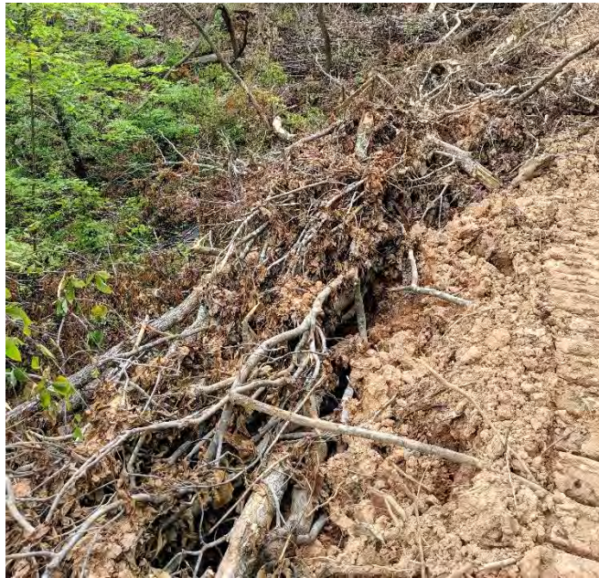
Figure 5U: A brush barrier alongside a skid trail
