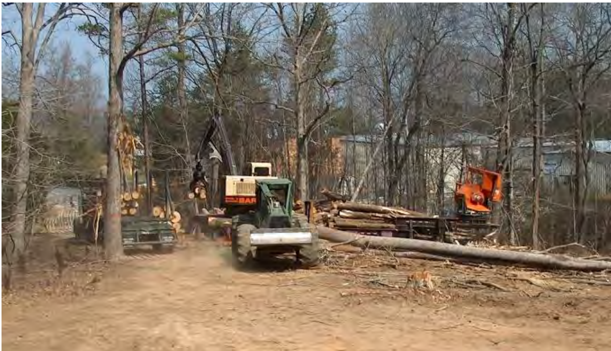
Figure 7-1: Active logging deck
