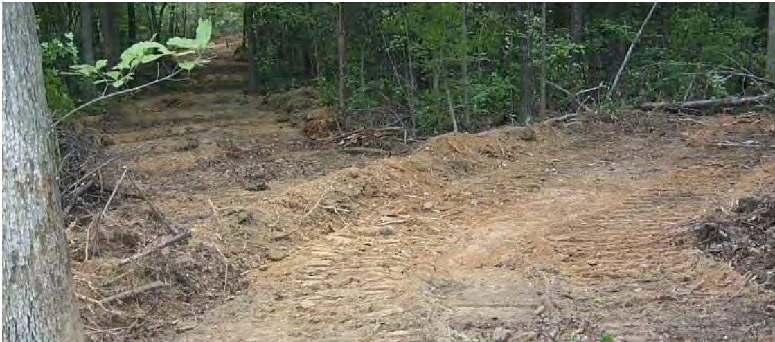
Figure 5G: A turnout used together with a waterbar on a skid trail
