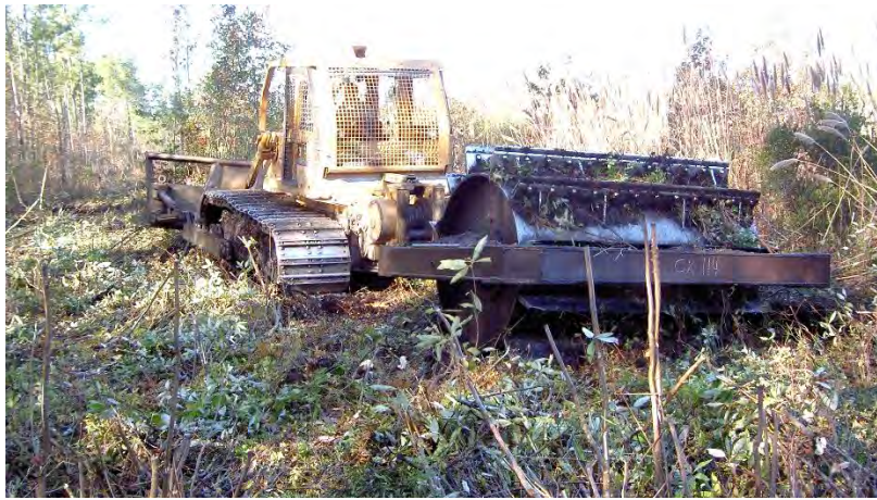
Figure 9D: Bulldozer pulling a drum chopper
