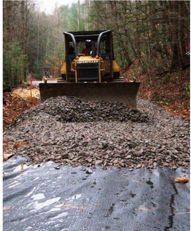
Figure 7E: Geotextile and gravel being applied atop a renovated legacy forest road
