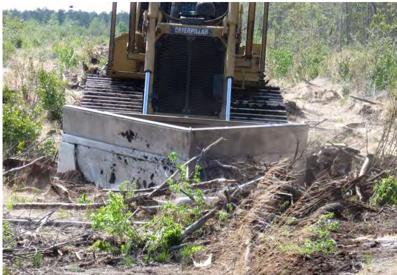
Figure 9F: Bulldozer with a V-blade pushing debris aside for bedding
