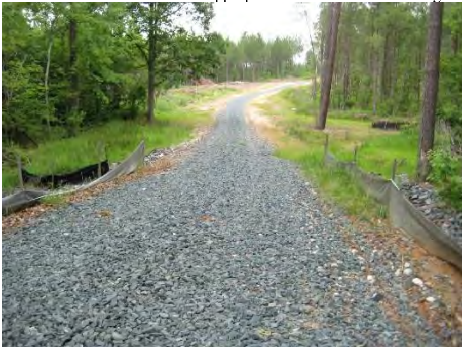
Figure 7A: A forest haul road built to a high standard
