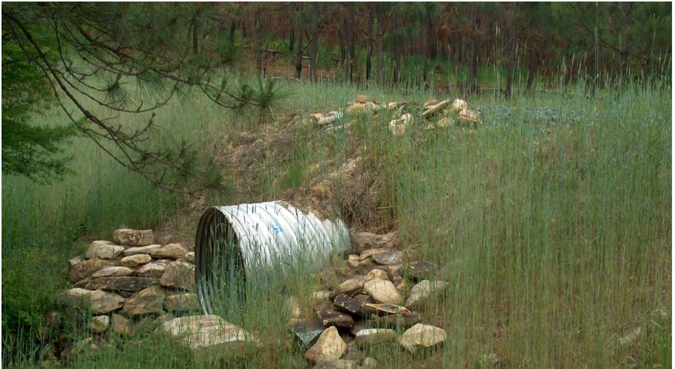
Figure 6D: Example of a permanent culvert stream crossing
