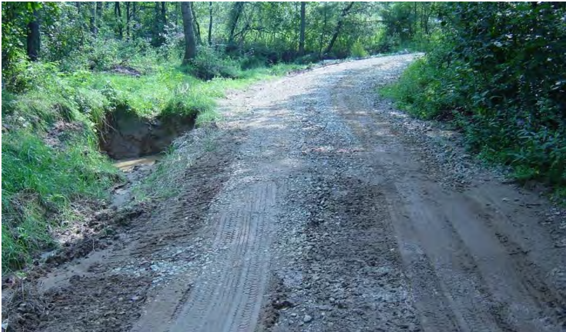
Figure 5O: Temporary sediment capture alongside a forest road Picture note: This temporary holding area, reinforced with stone, is successfully capturing runoff and sediment. The stone provides good support and backing.
