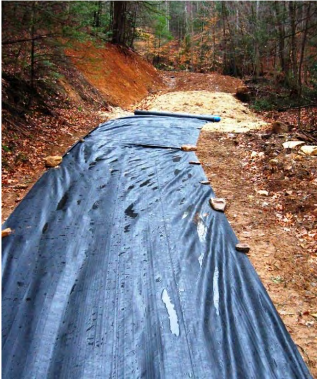
Figure 7E: Geotextile and gravel being applied atop a renovated legacy forest road
