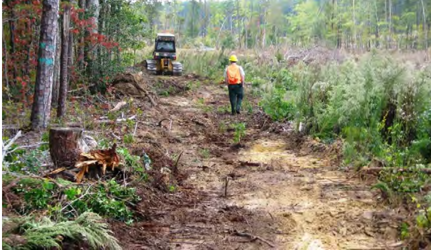
Figure 9B: A well-done bladed fire control line for a site prep burn
