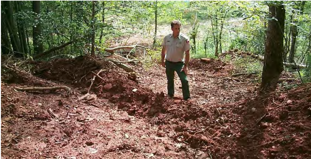
Figure 5C: Waterbar constructed across a skid trail
