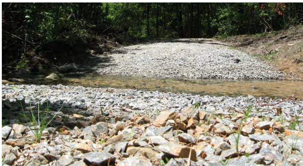
Figure 6O: Ground-level view of a newly installed ford
