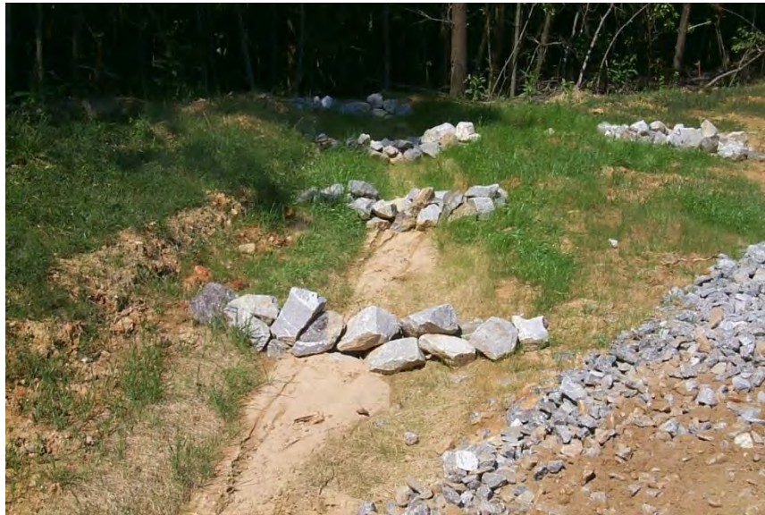
Figure 5V: Check dams installed within a turnout from a forest road
