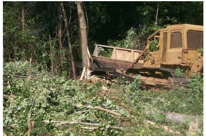
KG-blade used for shearing during site-prep.
