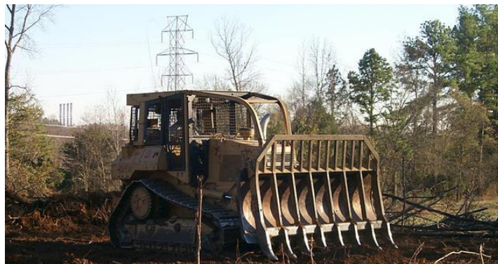
Root rake used to pile debris for site prep.
