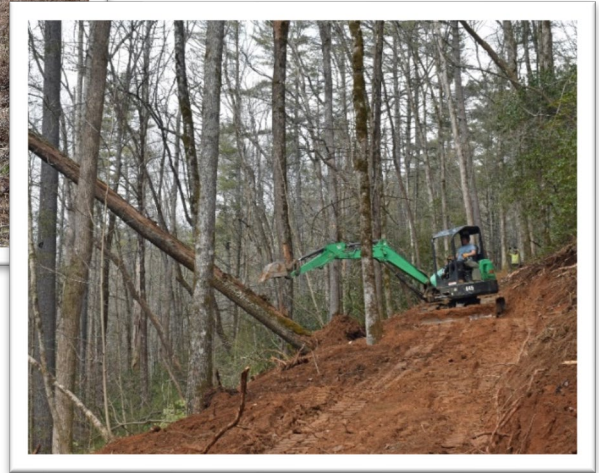
Trail construction near Hooker Falls
