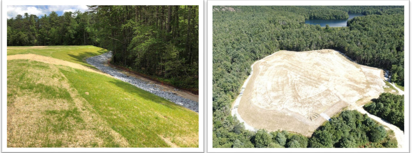
Figure 13: Solid Waste Management Unit 11 with reshaped banks and new landfill cap
