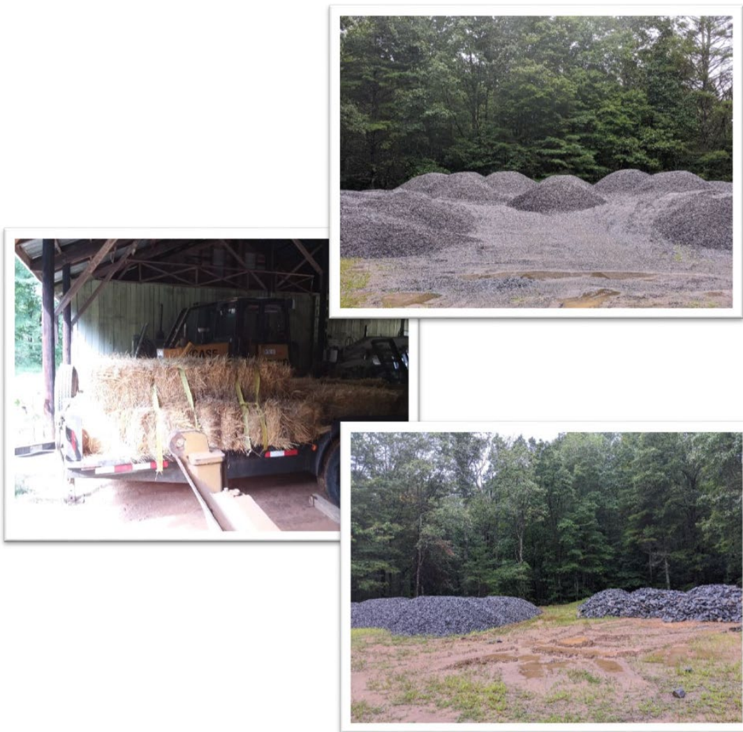
Figure 17: Gravel and erosion control materials
