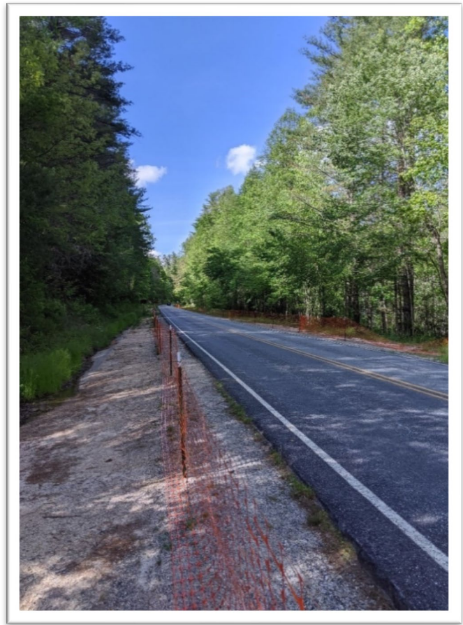
Limiting roadside parking along Staton Road with temporary fencing
