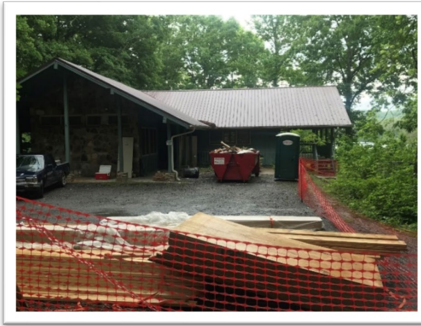
Renovation progress at Lake Julia office
