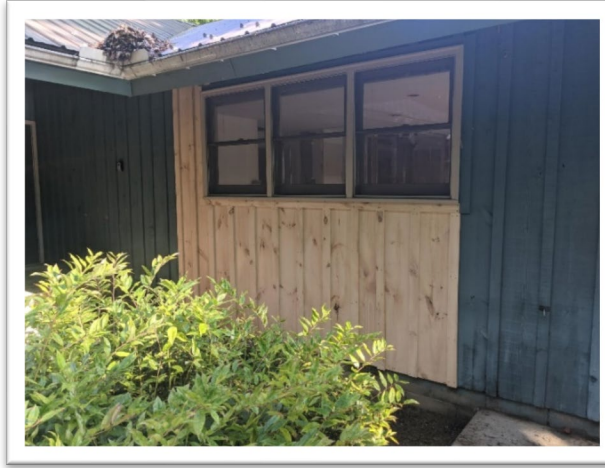
Exterior repairs to Lake Julia office
