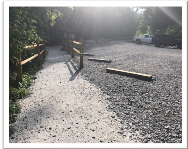
High Falls Access Area after improvements
