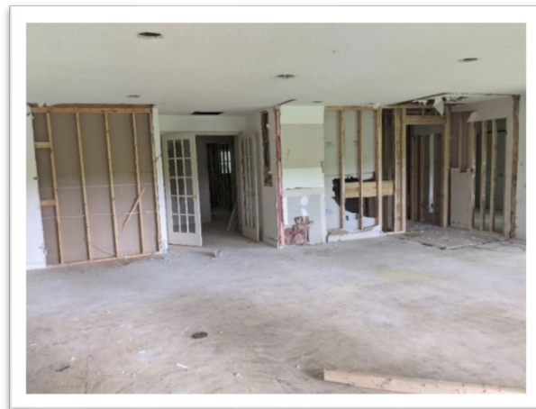
Interior remodel and mold remediation in Lake Julia office
