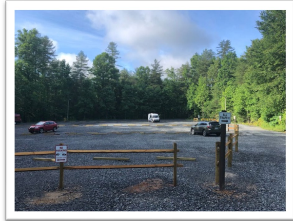
Lake Imaging Access Area after improvements
