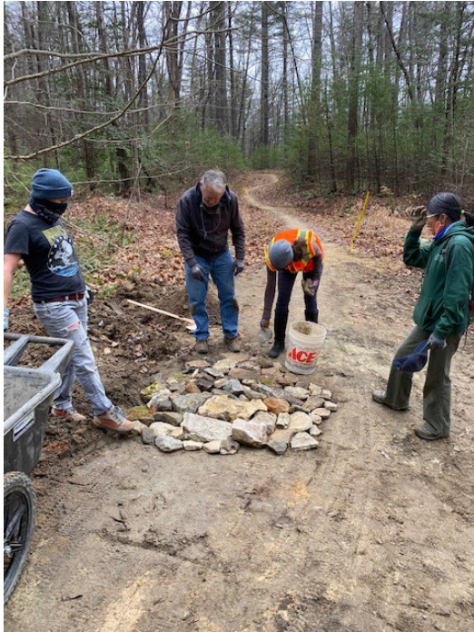
Volunteers use rock to reinforce a section of a trail.
