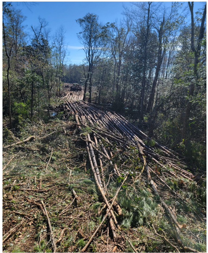
Figure 12. Skid trail log crossing. Correct: Skidder was able to move wood across the stream with no erosion issues. (Photo credit: Jason Harrell, PLM Logger).
