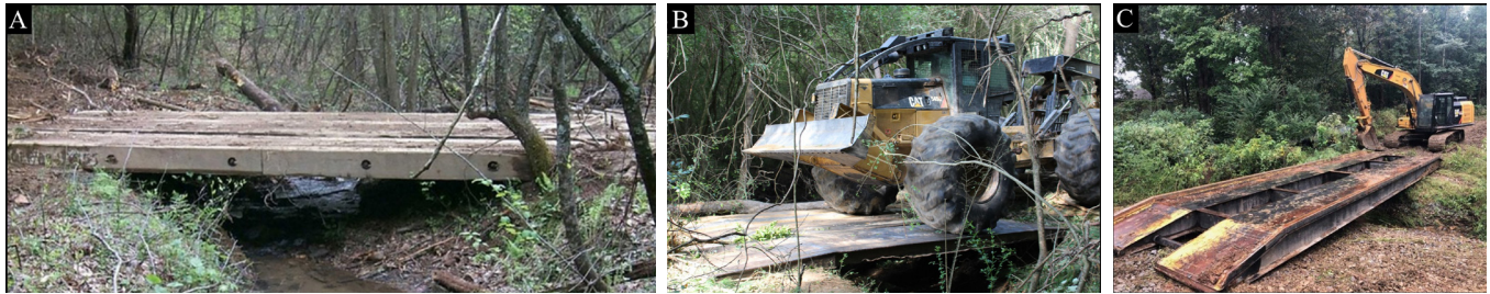
Figure 15. Portable bridge stream crossings: (A) wood panel, (B) steel panel, (C), steel bridge. Correct: - All good crossing methods. (Photo credit for A and B: North Carolina Forest Service)
