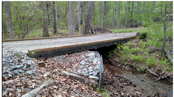
Figure 10. Forest road bridge stream crossing. Correct: Rock on the approaches, gabions, and vegetation protecting the stream banks.
