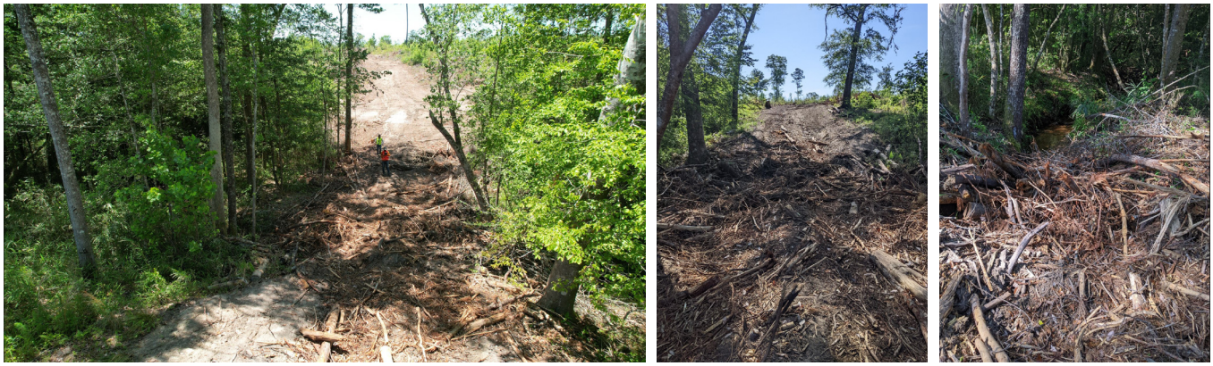
Figure 14. Logging slash and debris used for a skidder stream crossing. Incorrect: Never use logging debris and slash to cross a stream.
