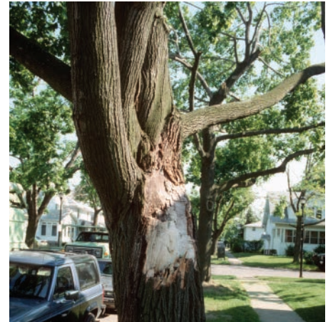
Scaffold branch loss exposing heartwood. Damage has occurred at the unions of other branches structurally compromising the unions. Remove tree. FEMA code F4.
