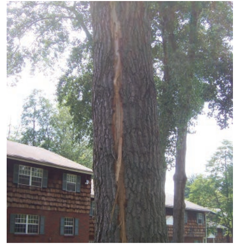
Lightning damage. Frayed bark associated with crack. Bark debris on the ground. Crack can run up to the top of the tree. If there is cracking into the heartwood consider removal. Have an ISA Certified Arborist inspect the tree. Potential FEMA code F4.
