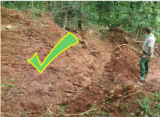
Waterbar is angled to divert runoff in a controlled manner.
