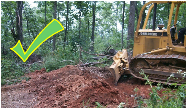
Start working from the uphill side, mounding the waterbar.
