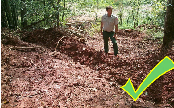
Waterbar is mounded and extends the full width across.
