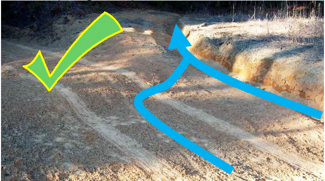
A rolling dip on the road diverts runoff into this wing ditch.
