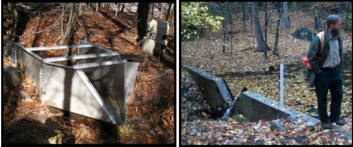
Figure 8. A flume and automated water sampler (left picture). A weir on the outlet of HFW1 (right picture).
