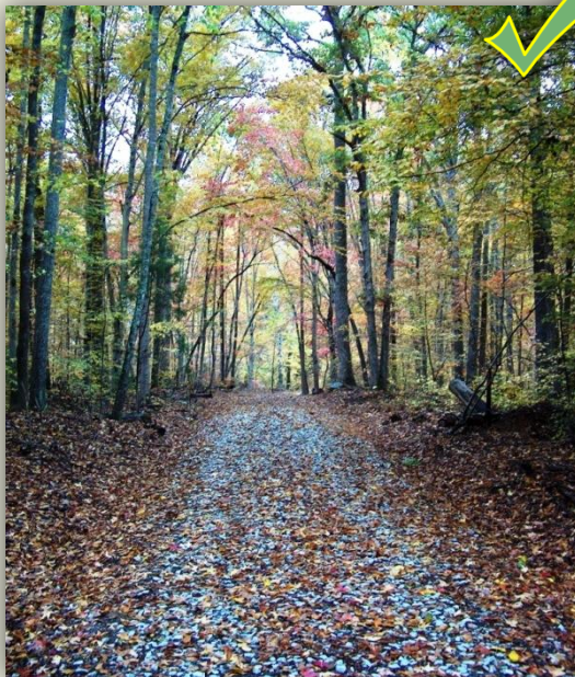
This forest access road is well maintained and has a stable surface of crushed stone that helps to control runoff.
