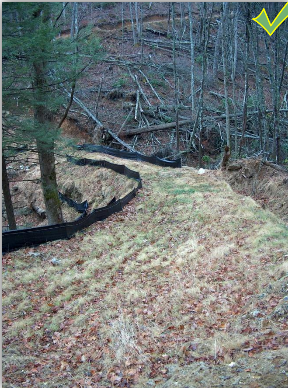
These pictures show well implemented BMPs for rehabilitation along skid trails in the Mountains. In both examples, the ground was seeded and mulched. Silt fence was installed as needed to slow runoff and reduce erosion.
