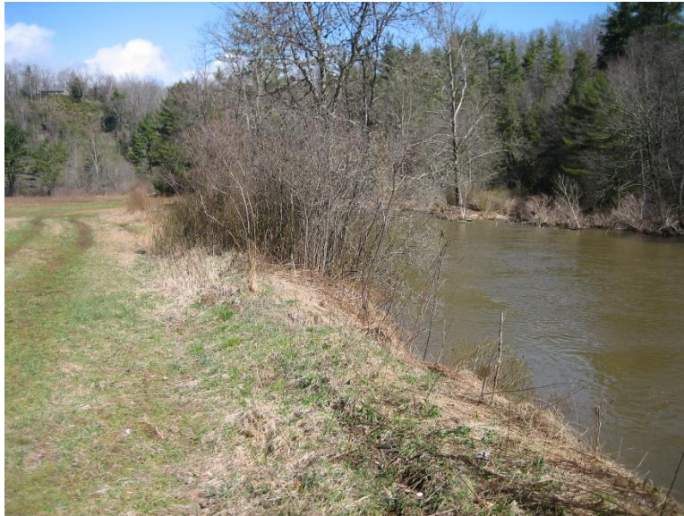
Photo 1: Reach 1, downstream view from adjacent field
