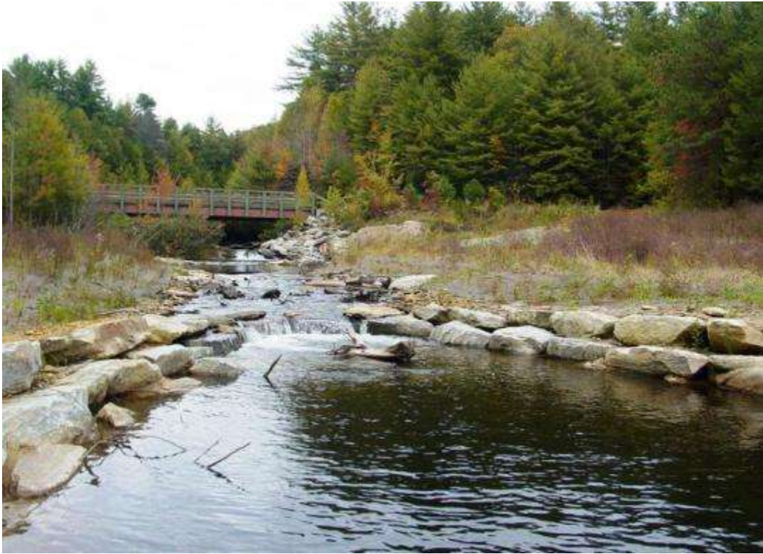
Above: Photo from October 2011. View looking upstream at one rock vane structure and its pool.
