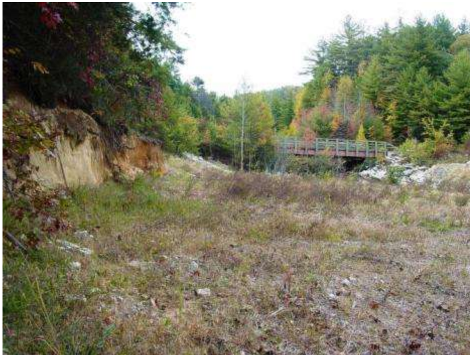
Photo October 2011. View looking upstream at location of former channel, against the backfilled embankment.
