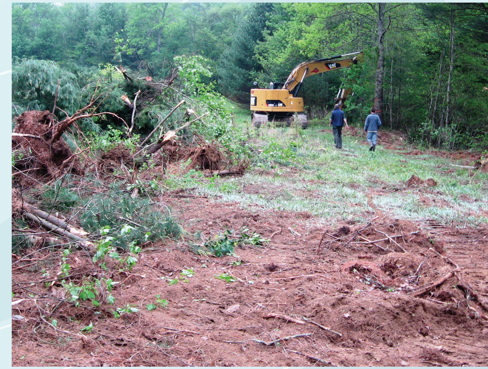
Surveying & clearing a new stream path.
