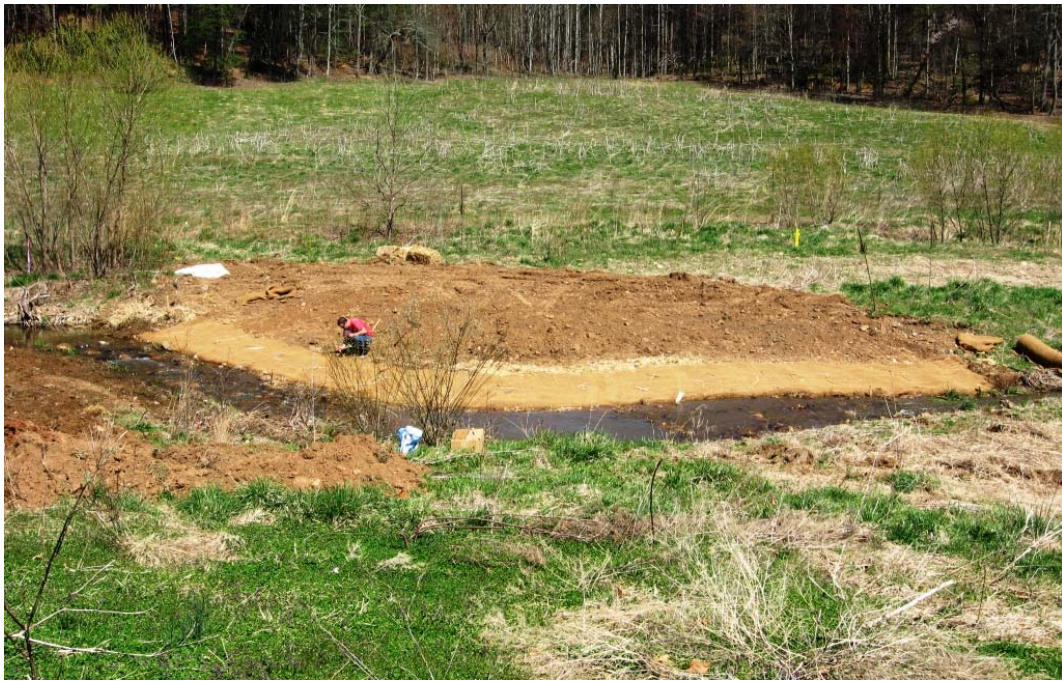
Photo 5: Overview of the stream repair work, April 2010.
