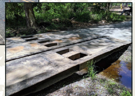
Right: Bridgemats on a logging job near the town of Marks Creek
