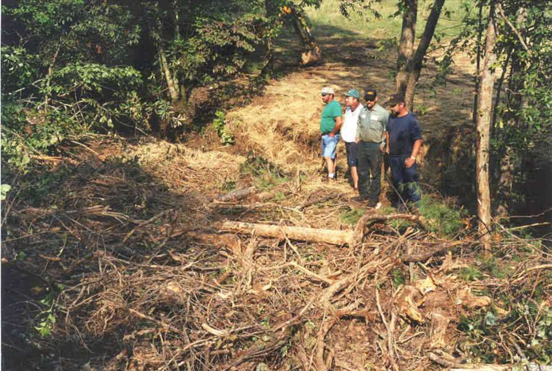
Another stream crossing stabilized, with slash & straw.
