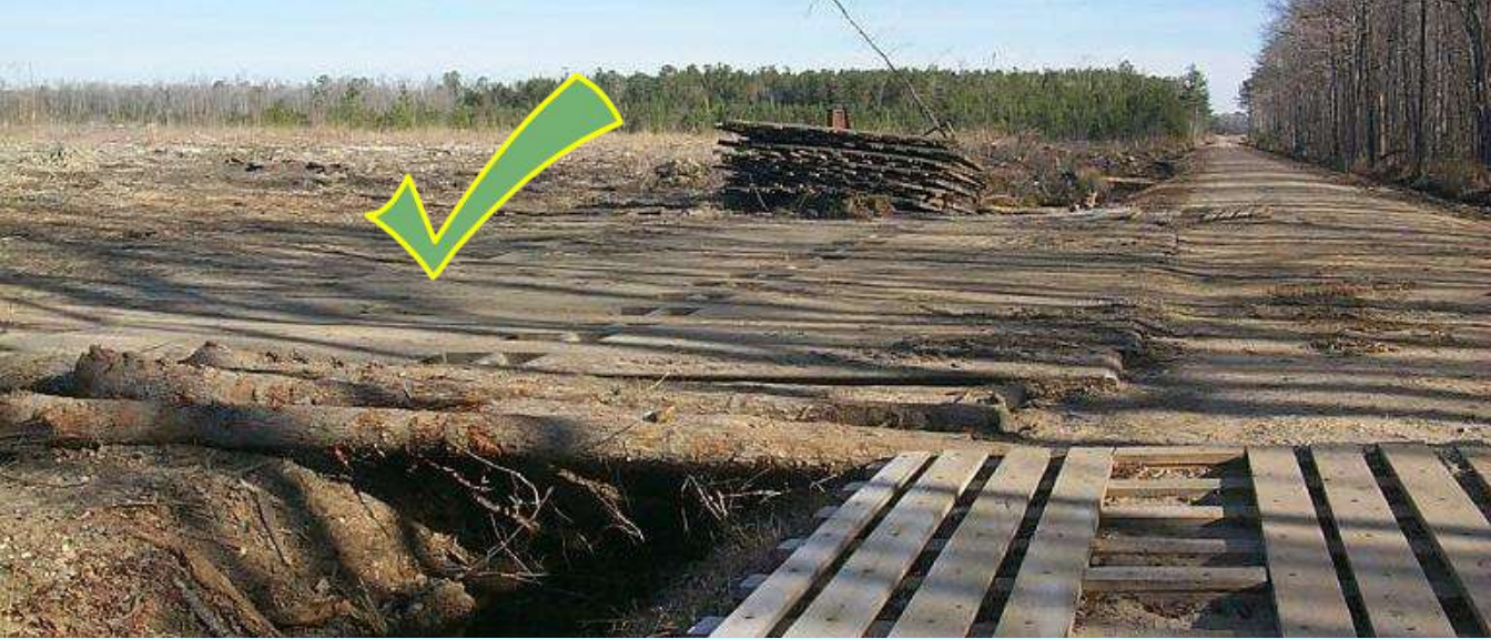
Bertie Co, ditch road crossing
