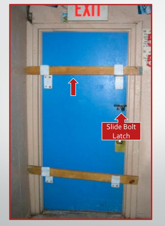
Wood or bars across an exit door while the building is occupied does not meet the requirements of 1910.36(d)(1). Nor does the closed slide bolt latch.
