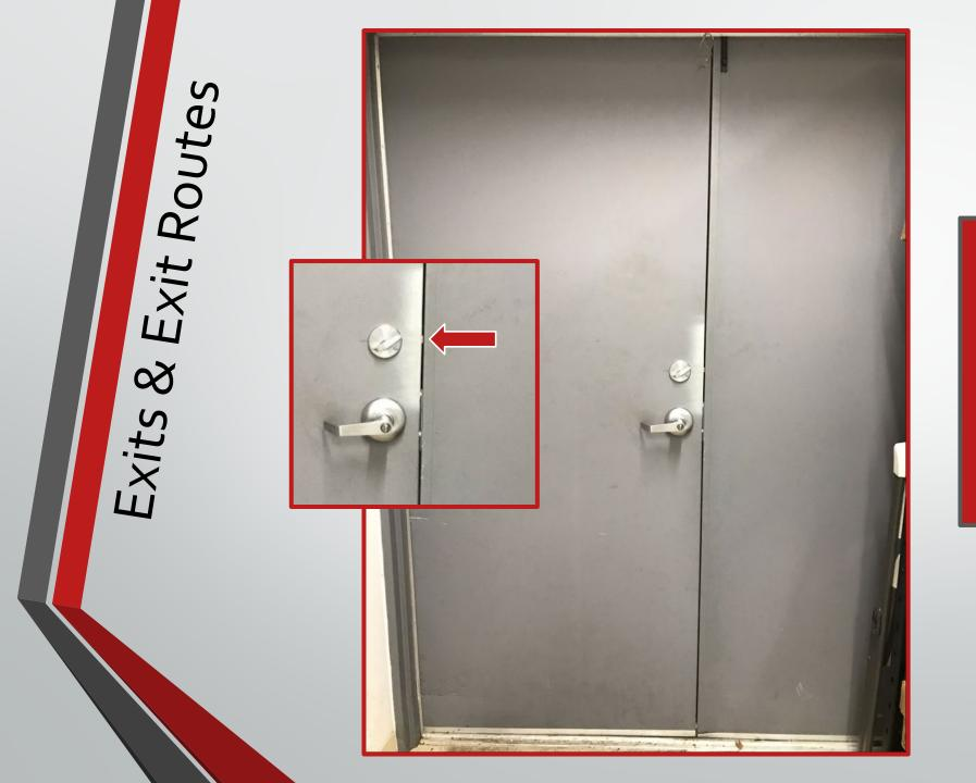
The deadbolt is locked, therefore the door does not meet the requirements of 1910.36(d)(1).
