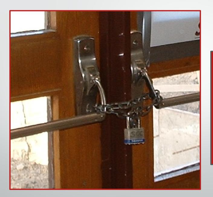
The chain with padlock on the door does not meet the requirements of 1910.36(d)(1) if the build is occupied.
