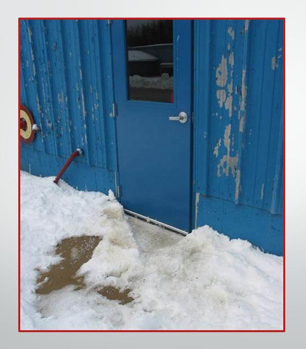
The exit door on the outside is obstructed by snow. This does not meet the requirements of 1910.37(a)(3) Exits & Exit Routes
