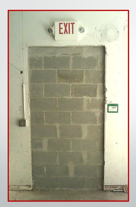
The exit doorway is obstructed by a wall. Some establishment will seal off exits when adding additions on. This does not meet the requirements of 1910.37(a)(3)
