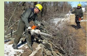
Chain saw crews working after winter storm
