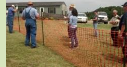
Temporary Fencing by AERT Team
