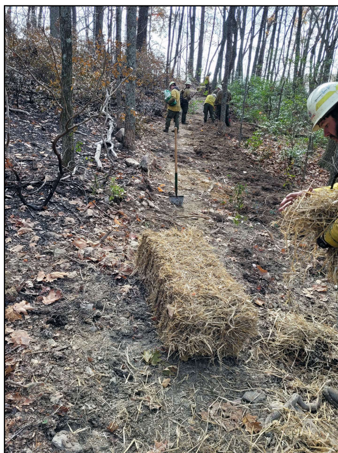
To prevent accelerated water runoff and soil erosion, ground personnel are using grass seed and straw to stabilize the fire lines, especially in steep terrain and near and around intermittent and perennial streams.
