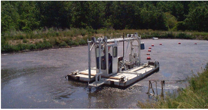
Figure 3. Sludge dredging in a waste lagoon (Source: Closure of Earthen Manure Structures [Including Basins, Holding Ponds and Lagoons]. 2006. Animal Agriculture and the Environment: National Center for Manure and Animal Waste Management White Papers )
