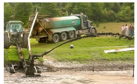
Figure 2. Lagoon sludge agitation and pumping (Photo courtesy of Rutland Herald)
