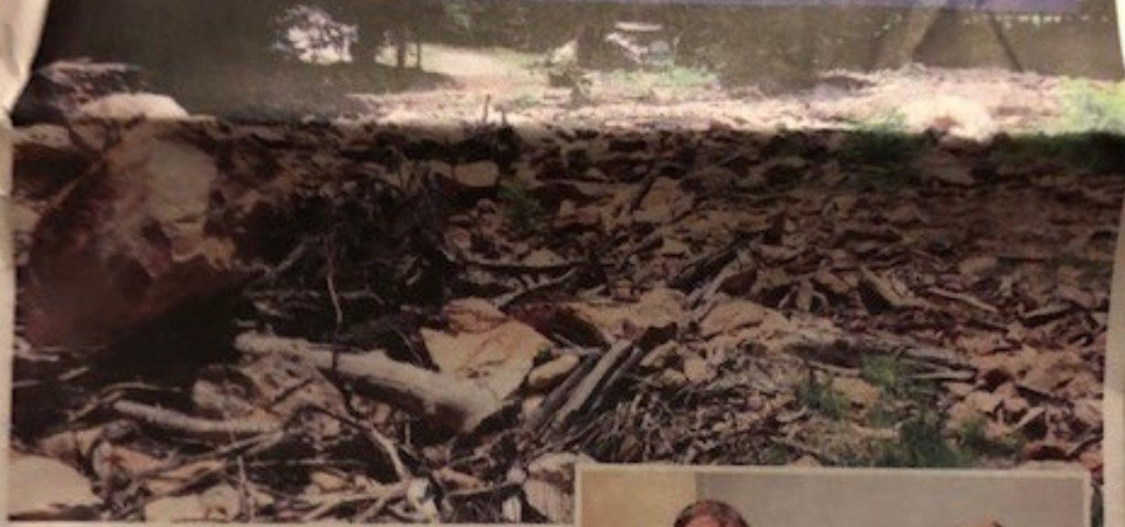
MASSIVE OBSTRUCTIONS — This stream bed photo shows the massive obstructions still clogging the East Fork of the Pigeon River.
