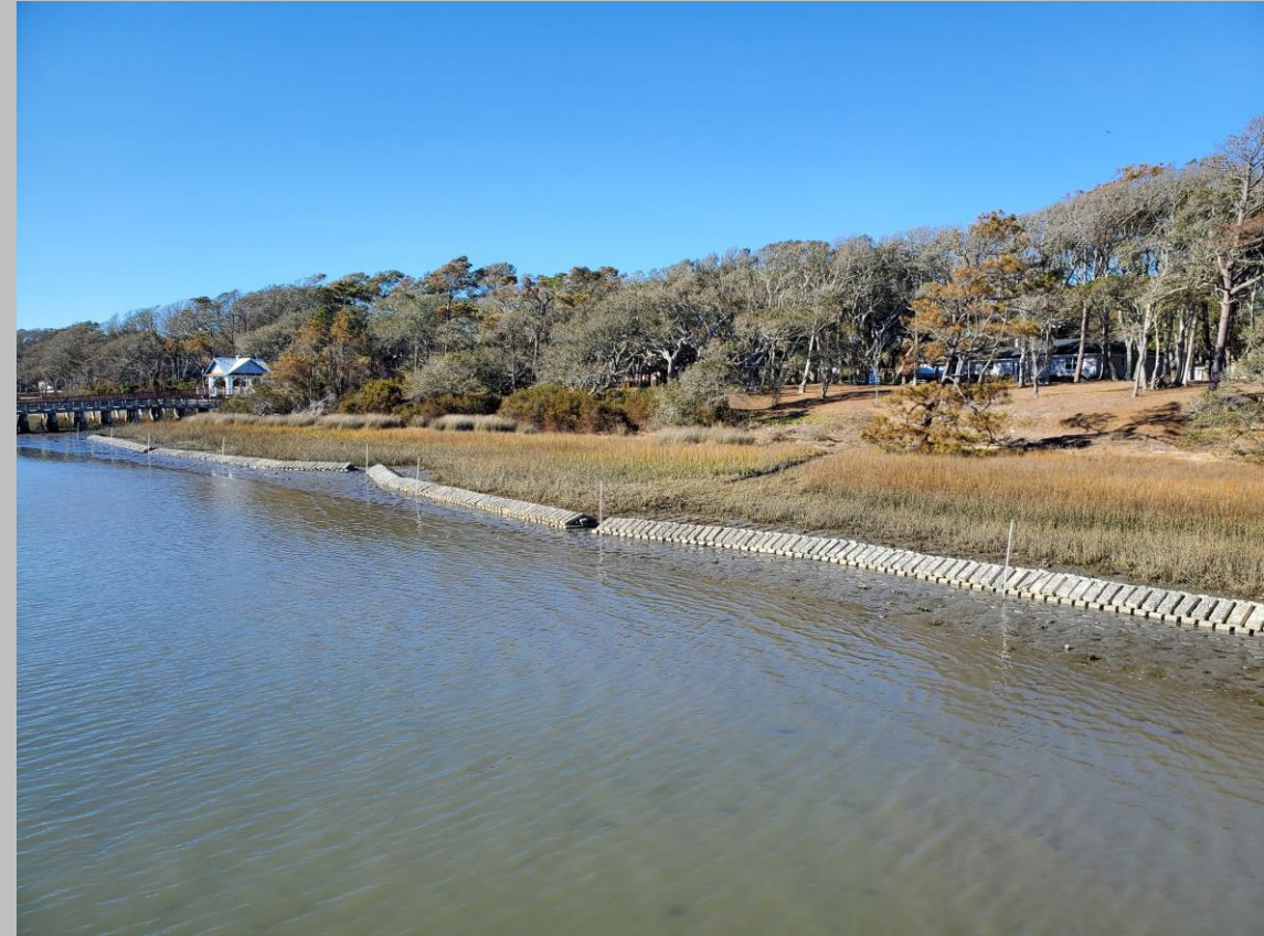
Photo at low tide showing placement of the breakwaters/sills on the landscape
