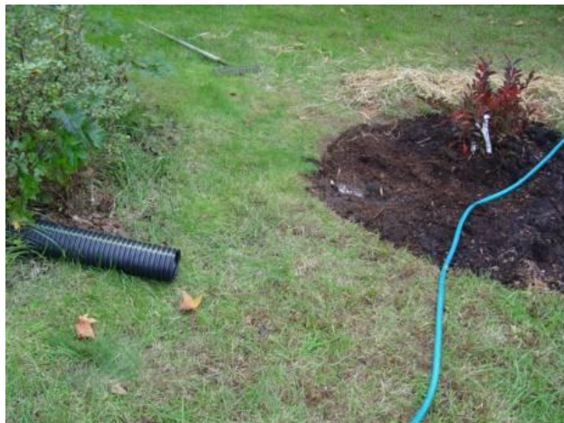
Figure 5.6 Stormwater flowing across flat, grassed slope before entering a rain garden.
