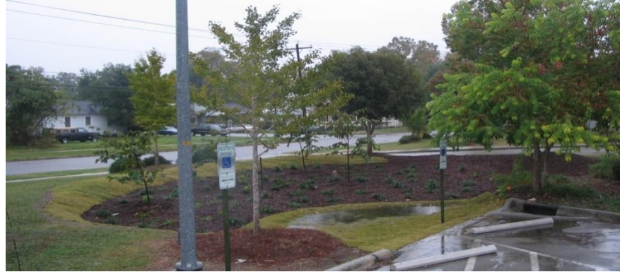
Figure 5.7 Rain garden in Wilmington, NC with a small forebay.
