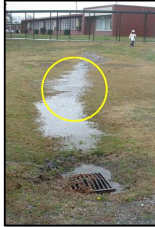
Figure 5.3 Locate rain gardens between the runoff source and its destination (an existing storm drain).
