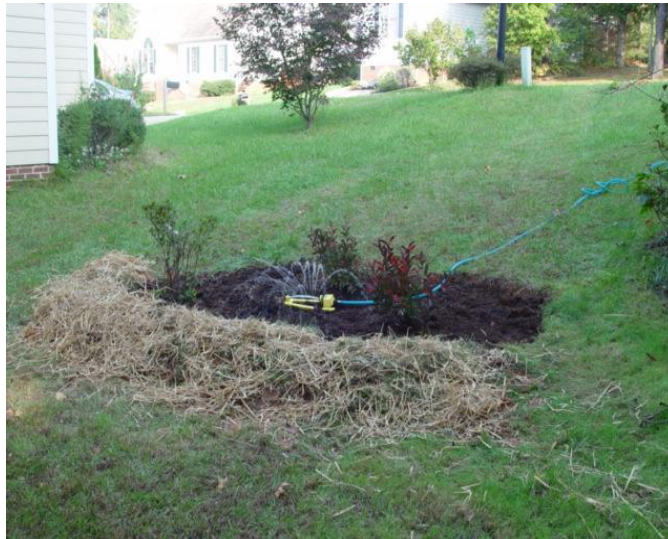
Figure 5.10 Earthen weir immediately following installation.
