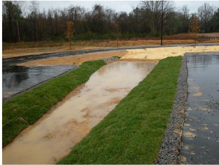
Figure 5.8 Examples of a gravel verge and vegetated filter strip receiving sheet flow from a parking lot.
