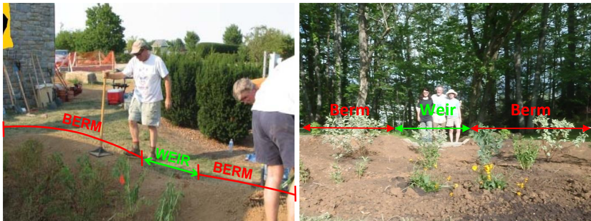
Figure 5.5 Examples of a berm and a weir in a backyard stormwater practice.
