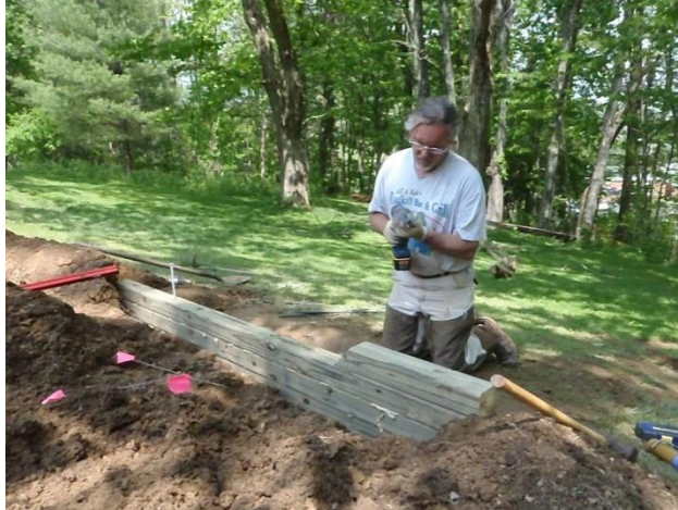
Figure 5.9 An example of a wooden weir installation.
