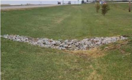
Figure 6.4 Swale with check dam constructed of stone. (Source – USDA – Natural Resource Conservation Service – Illinois)
