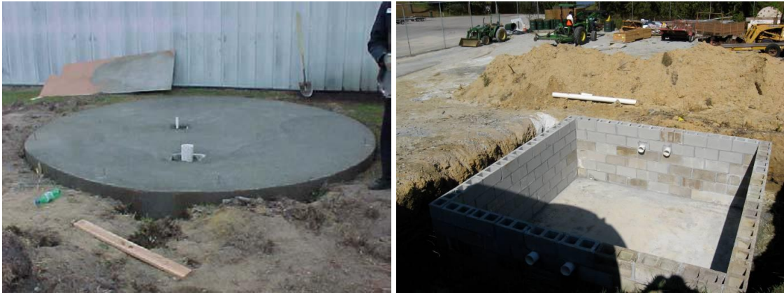
Figure 7.16. Concrete pads constructed to support cisterns greater than 1,500 gallons.
