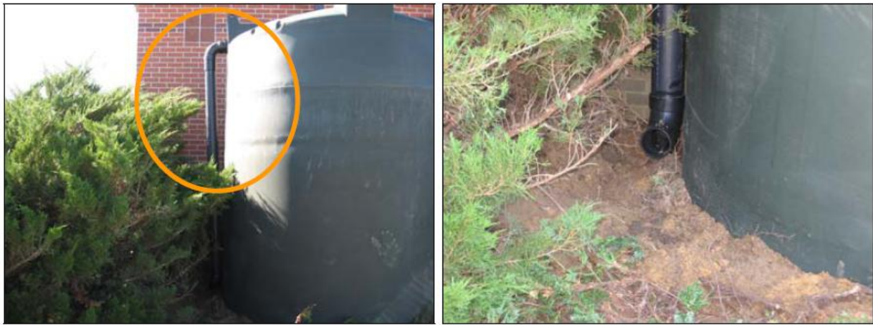
Figures 7.13 and 7.14 Overflow assembly on cistern.
