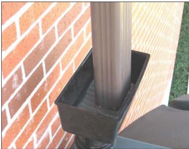
Figure 7.12 Debris filters just below gutter downspout.
