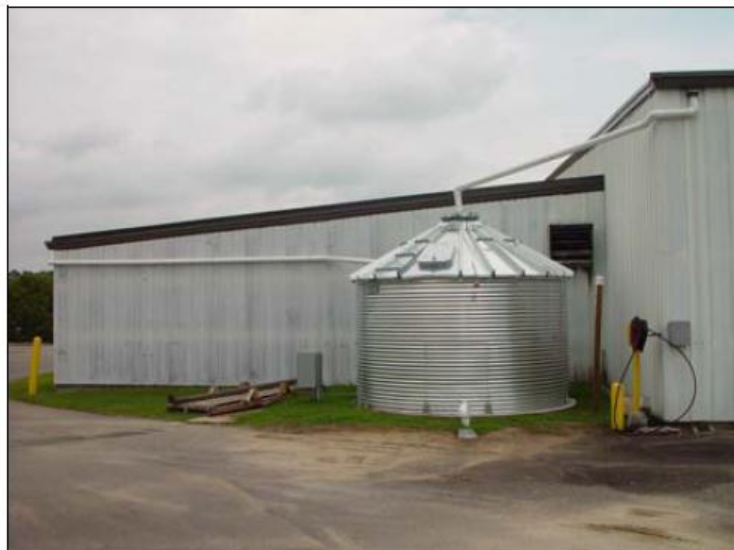
Figure 7.1 3,000-gallon cistern installation in Greenville, N.C.
