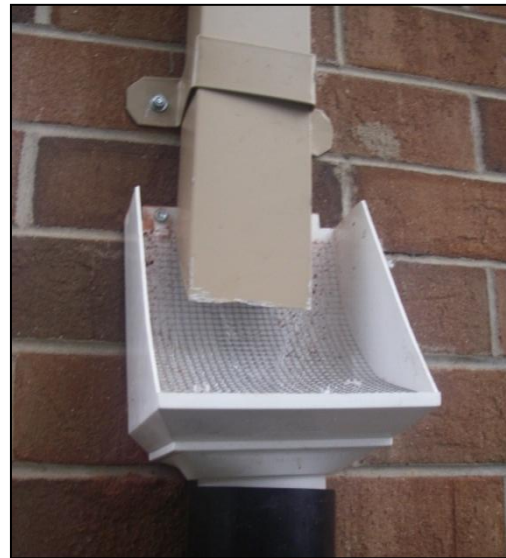
Figure 7.12 Debris filters just below gutter downspout.
