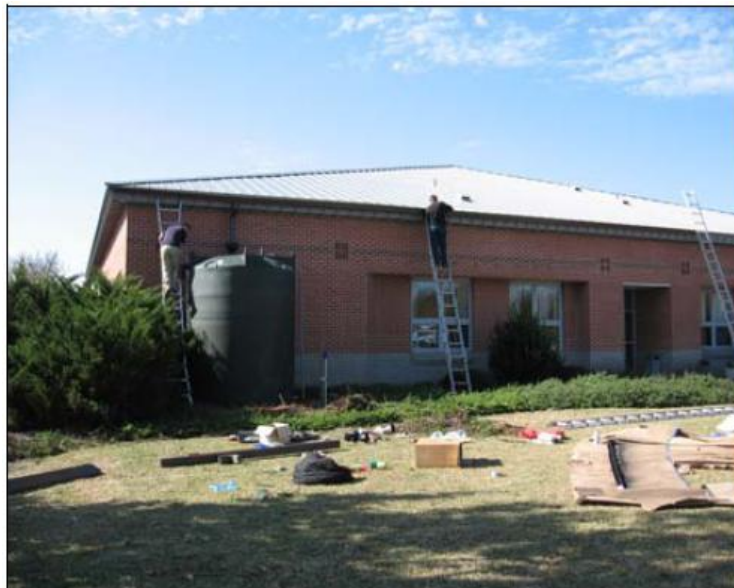
Figure 7.1 3,000-gallon cistern installation in Greenville, N.C.
