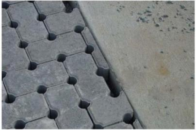
Figure 10.5 Pavers abutting a concrete edge.
