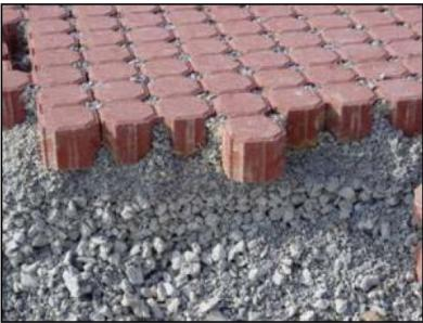
Figure 10.6 Gravel layers under permeable pavers.
