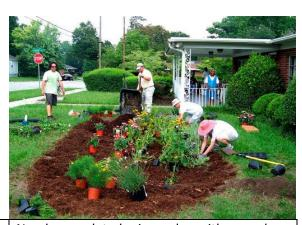
Nearly completed rain garden with a good layer of proper mulch and plant material selection. As this is not quite completed, any areas of heavy mulch layers (such as at the forefront of the photo) can readily be raked out for the proper, consistent layer.
