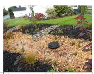
The vegetation is minimal on this site. While newly planted and immature, even when fully grown the spacing for this garden is not optimal. Care should also be taken on the cobble drainage coming into the garden for potential erosion and sedimentation. Note the mulch, it is too course and will likely lead to flotation, potentially filling the drop inlet (the black grate in the center) with debris
