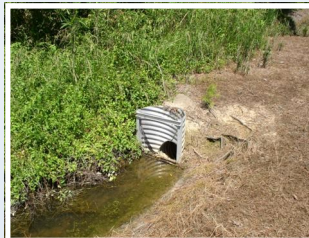
Water control structure
