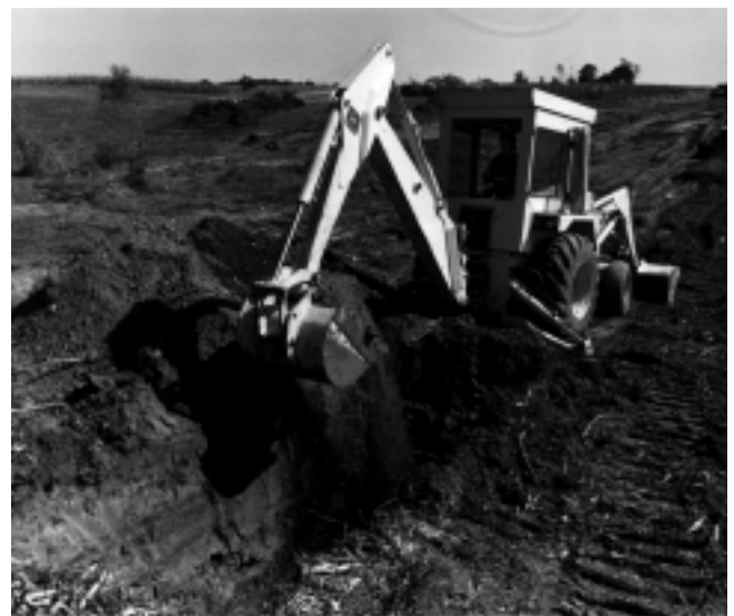
Figure 27 A core trench is cut on the centerline of a dam
