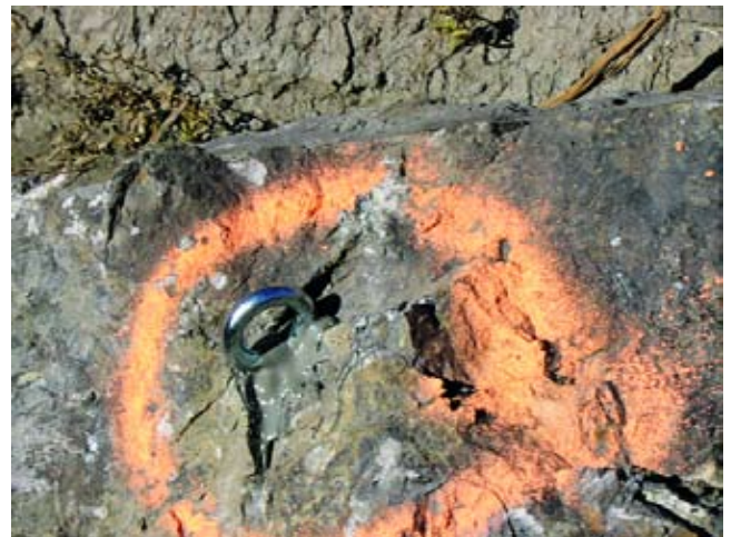
Figure TS14E-9 Eyebolt anchored in boulder with epoxy
